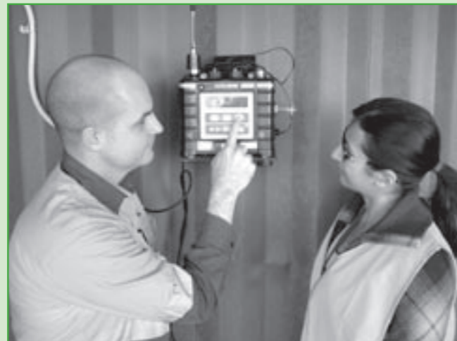
Above: Continuous VOC monitoring for air quality, 24 hours a day, seven days a week.
