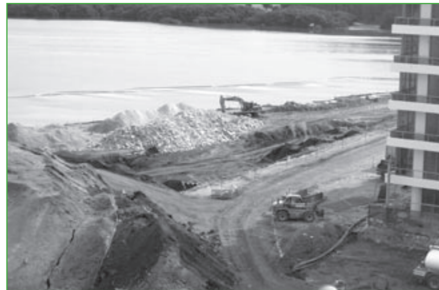
Backfilling treated soil on the Allied Feeds Project.
