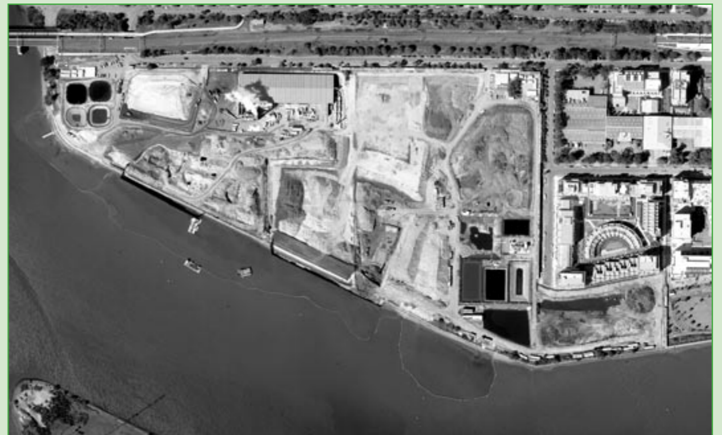
Above: Aerial view of the Rhodes Remediation Projects, March 2007.
