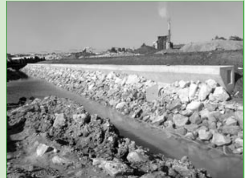
Above: Seawall construction, April 2007.
